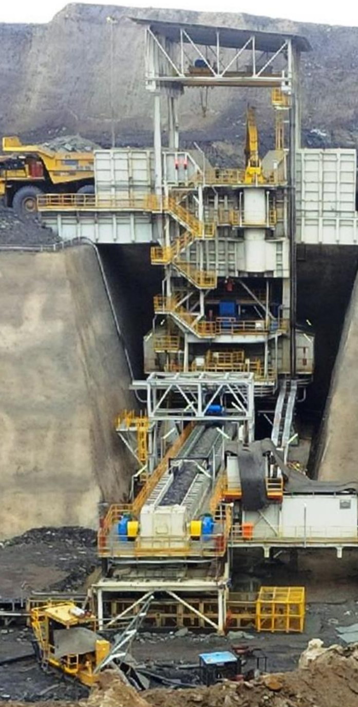
Semi-mobile in-pit crusher
