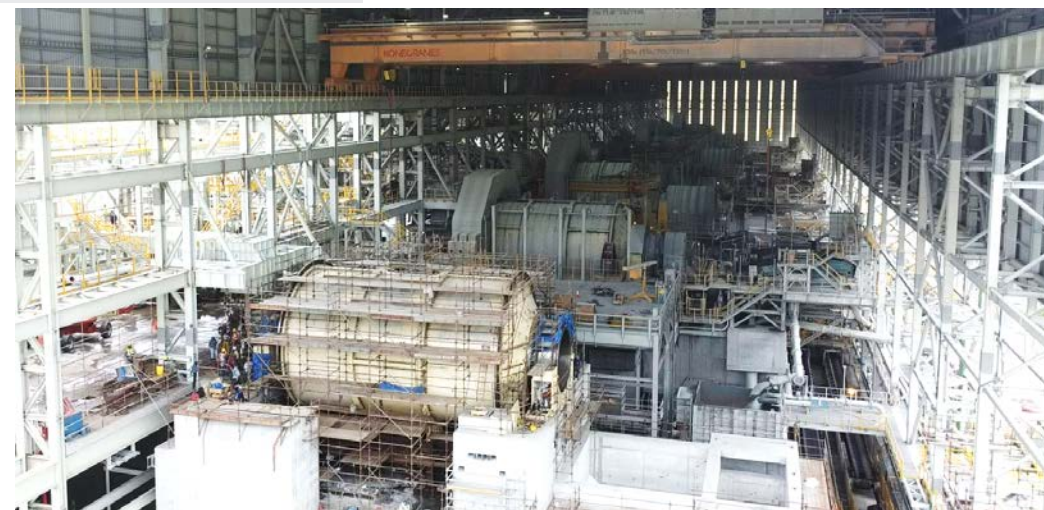
Ball Mill 6 Construction
