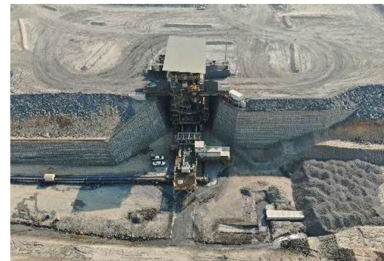
In Pit Crusher in Stage 3
