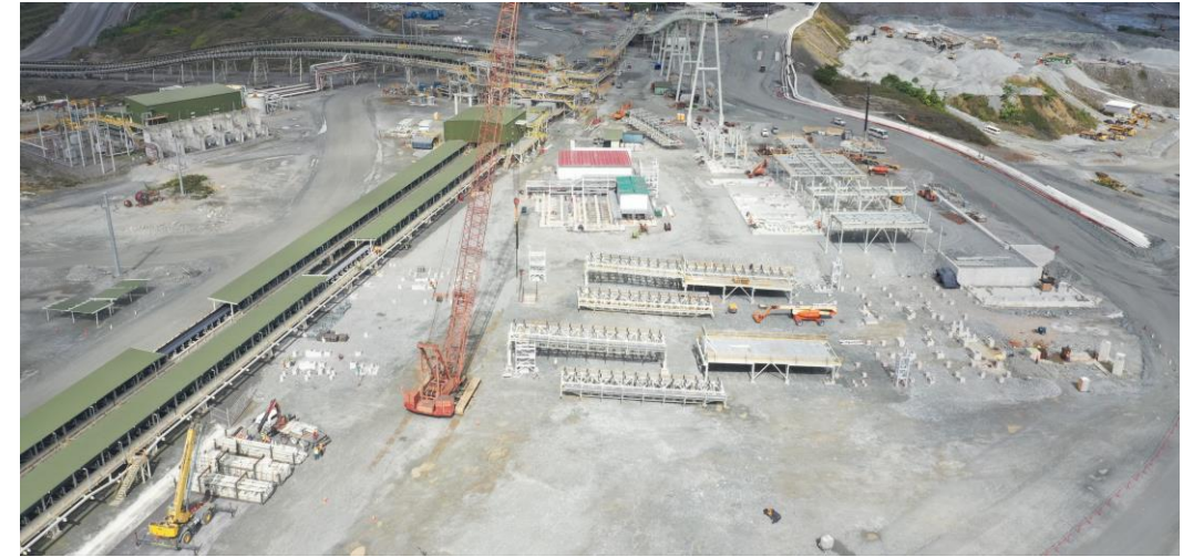
Screening Conveyors Progress
