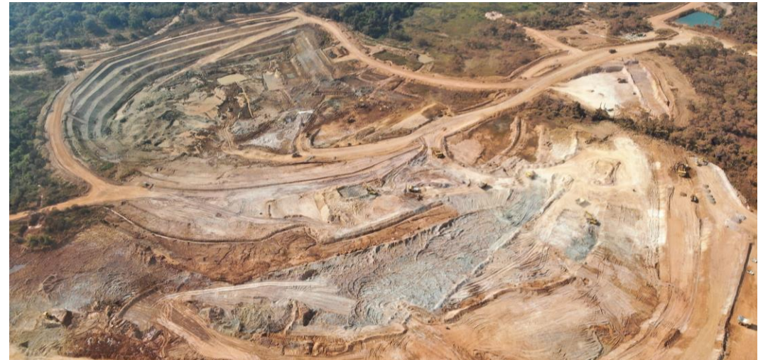
Aerial View of Enterprise Pit
