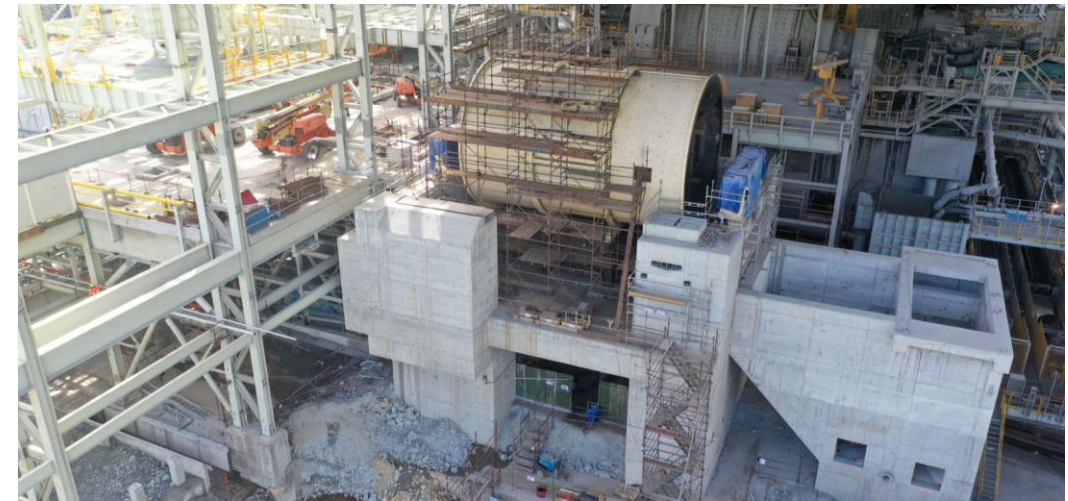
Ball Mill 6 Construction
