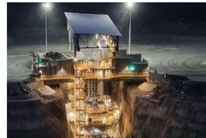
In-pit crusher at Sentinel
