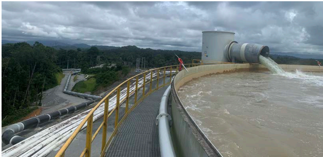
Decant Water Commissioning
