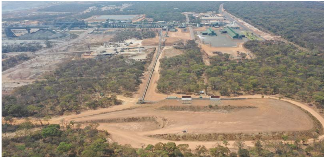
Ore Receiving Area and Crushing
