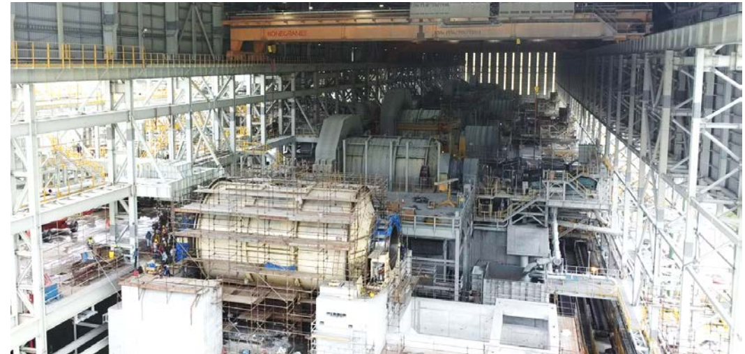
Ball Mill 6 Construction
