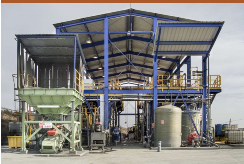
Las Cruces Poly Metallurgical Refinery Pilot Plant
