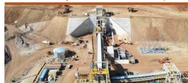
Sentinel Fourth In-Pit Crusher
