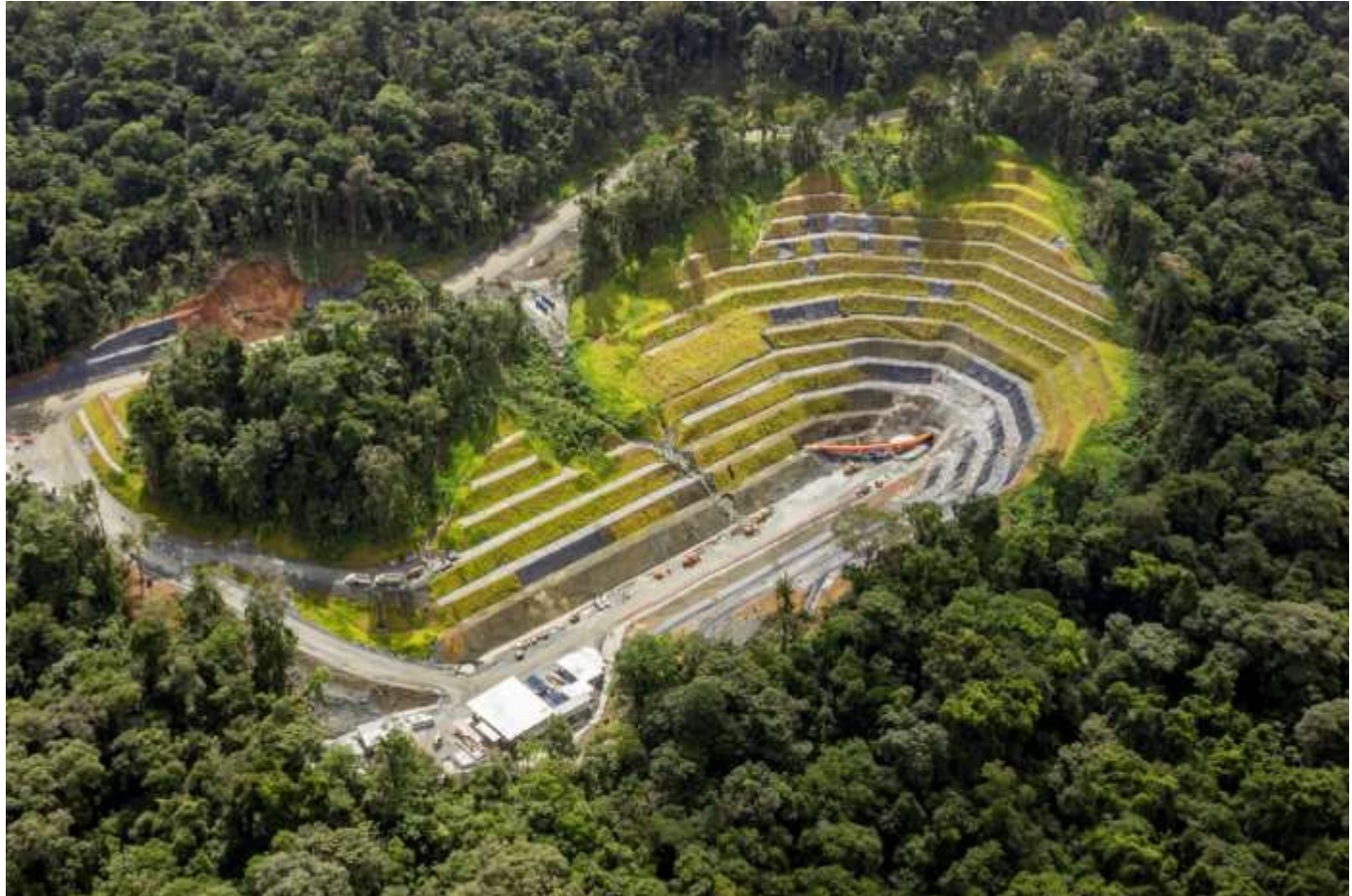
TMF DECANT OUTLET CHANNEL 01-FEB-2016
