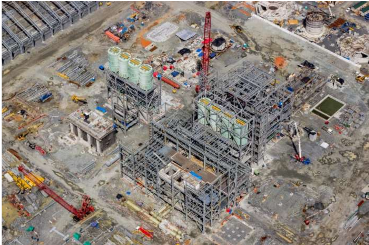
POWER PLANT UNIT 1 & 2 OVERVIEW 01-FEB-2016
