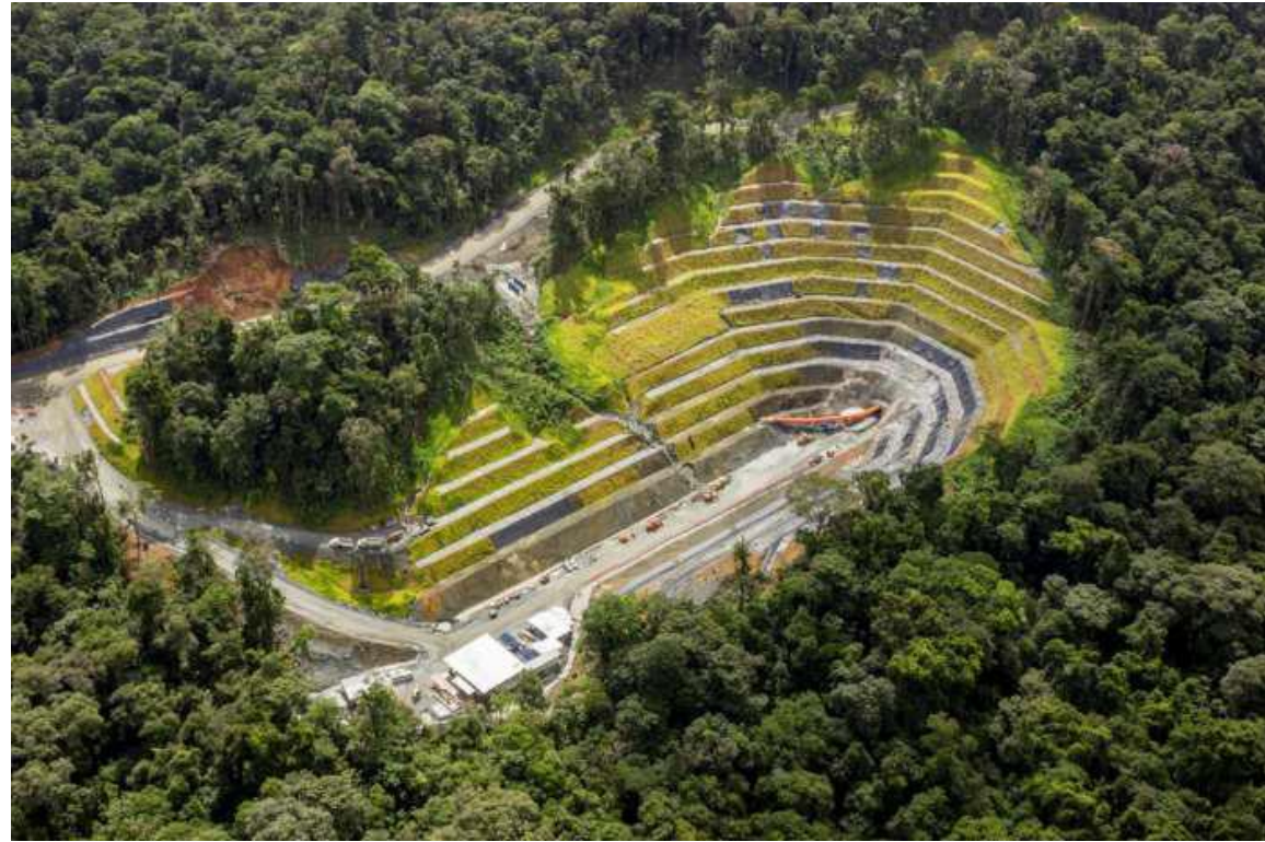
TAILINGS MANAGEMENT FACILITY DECANT OUTLET CHANNEL 01-FEB-2016
