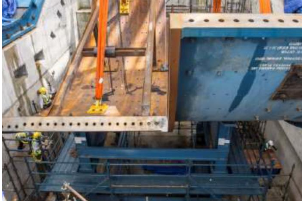
FIRST MILL SHELL INSTALLATION 10-FEB-2016
