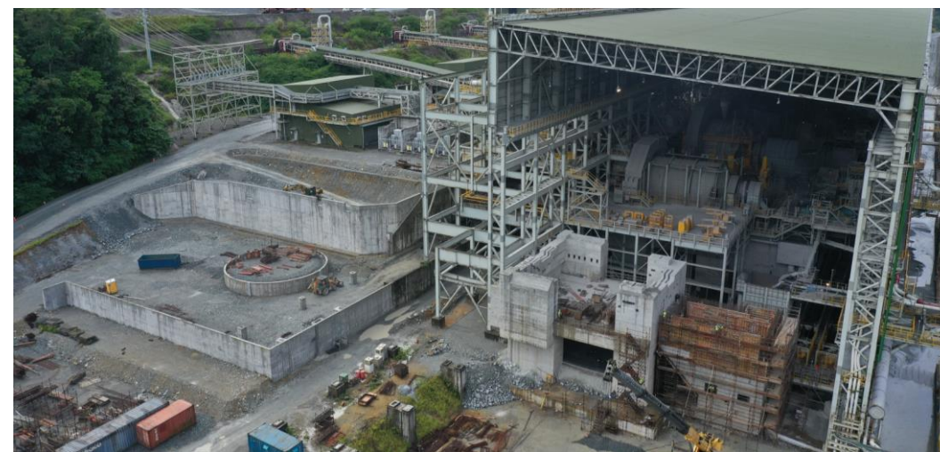
Cobre Panama Ball Mill 6 Progress
