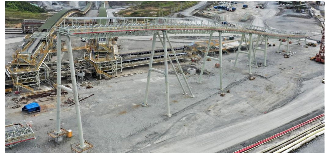
Screening Conveyors Progress
