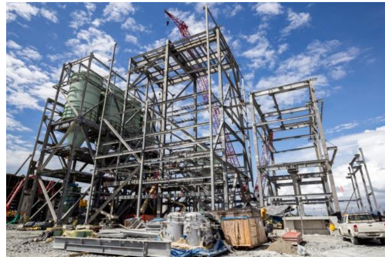
UNIT 1 BOILER & SCR STEEL
