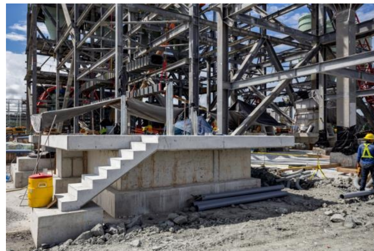
UNIT 1 FD FAN FOUNDATION – EAST SIDE
