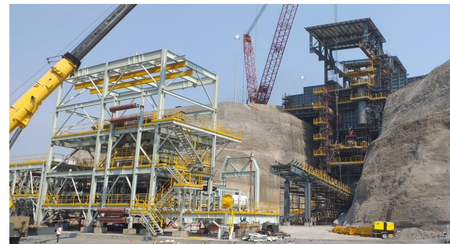
Sentinel Fourth In-Pit Crusher
