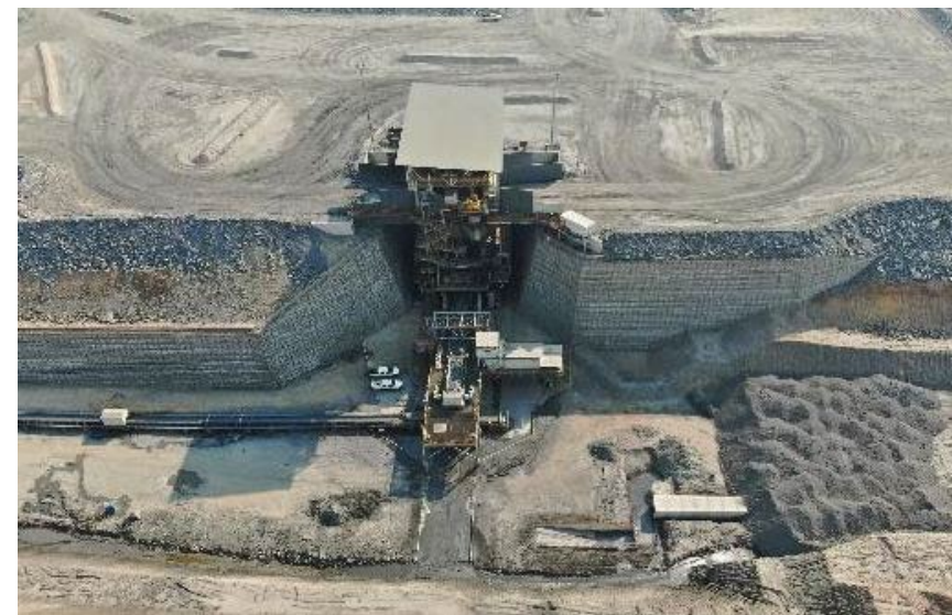
In Pit Crusher in Stage 3
