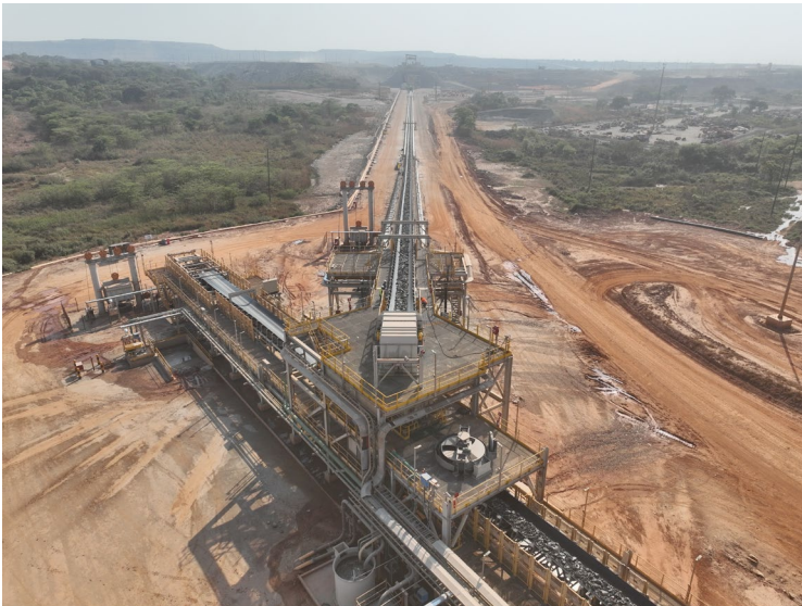
Stockpile Feed Conveyor
