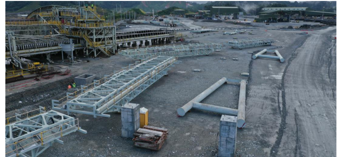
Screening Conveyors Progress
