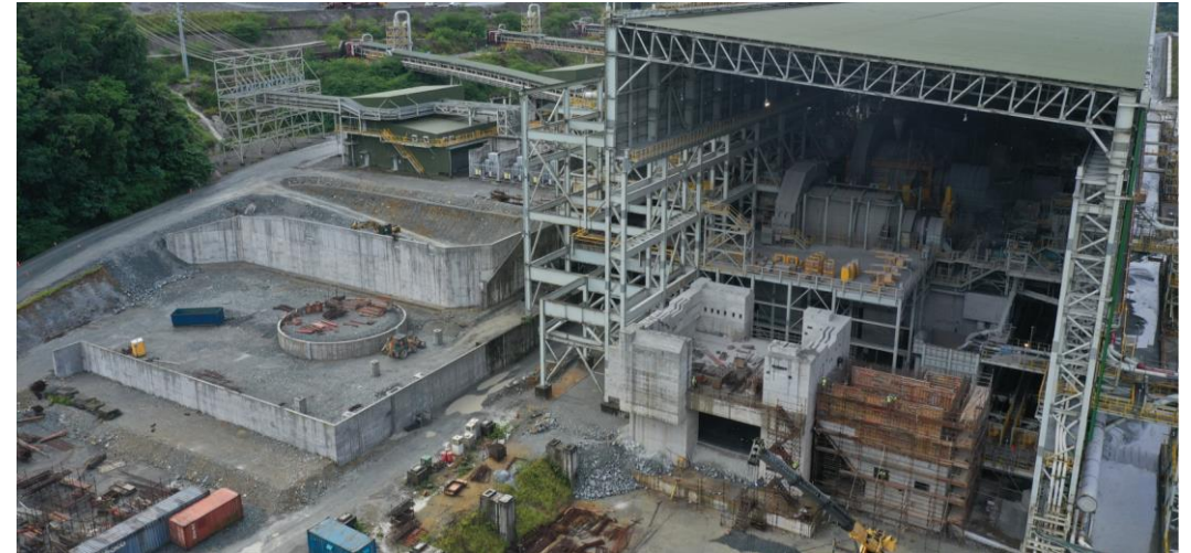
Cobre Panama Ball Mill 6 Progress
