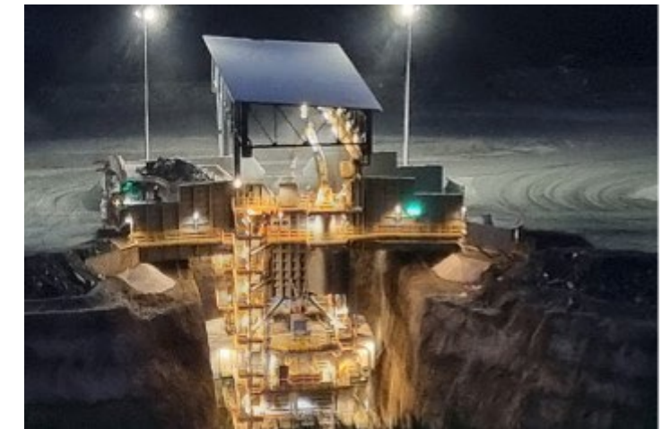
In-pit crusher at Sentinel
