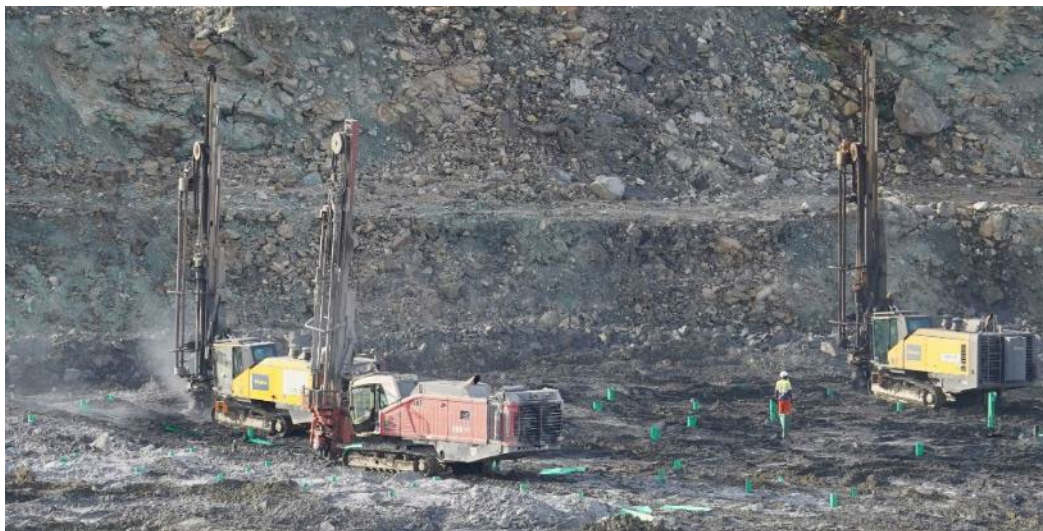
Drilling to blast
