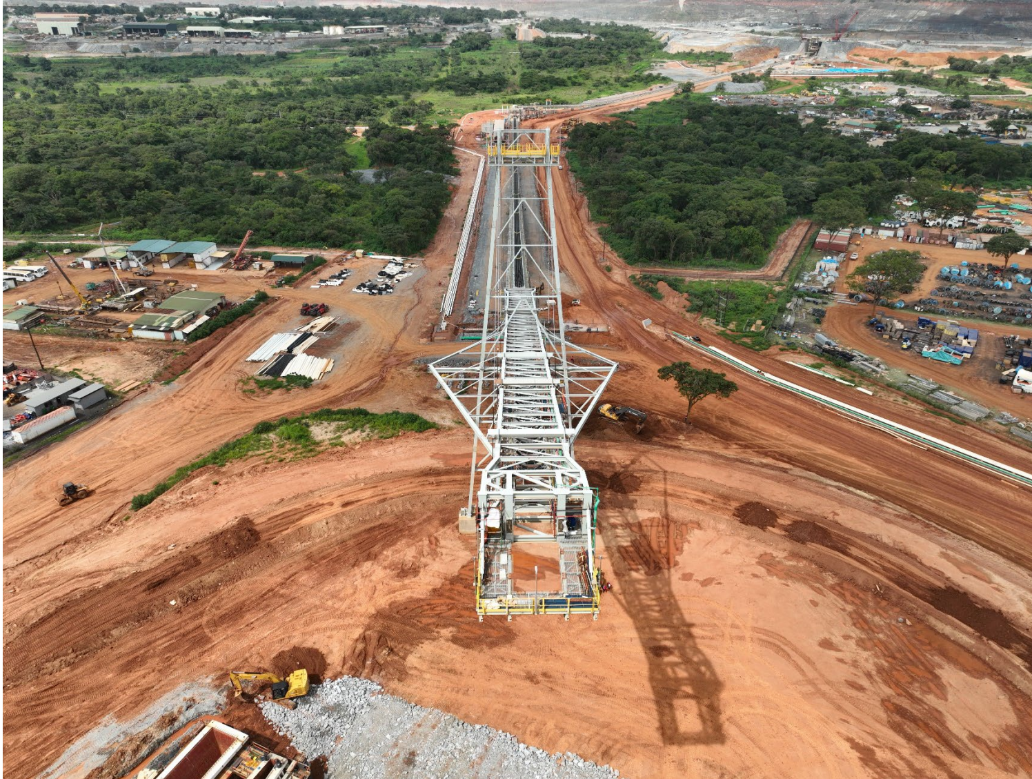
Stockpile Feed Conveyor with transfer station 2 in the middle and primary crusher in the back ground
