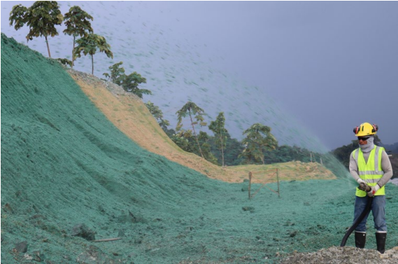
Hydroseeding at Cobre Panamá
