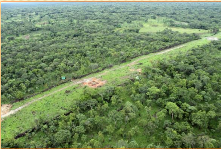
POWERLINE CLEARING & EARTHWORKS 20-DEC-2013
