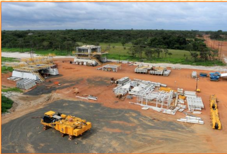
CRUSHER ASSEMBLY YARD 31-DEC-2013
