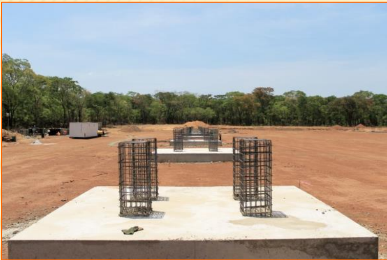
ABB SWITCHYARD, EAST GANTRY FOOTINGS 01-NOV-2013
