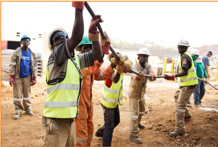
CABLE PULLING 31-DEC-2013
