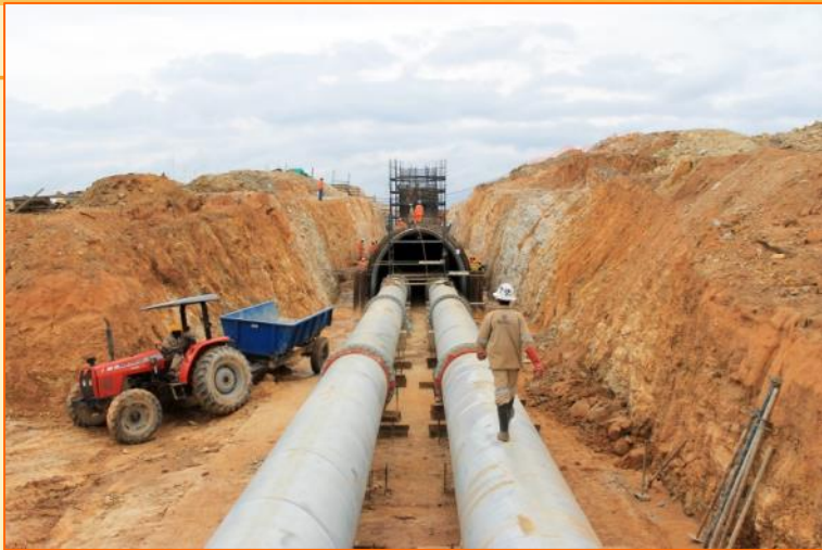
CHISOLA DAM, OUTLET PIPE & TUNNEL 2-JAN-2014
