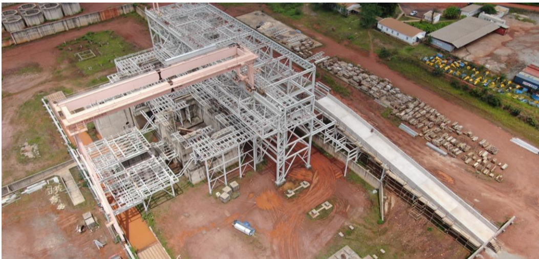
Concrete Mill Ramp
