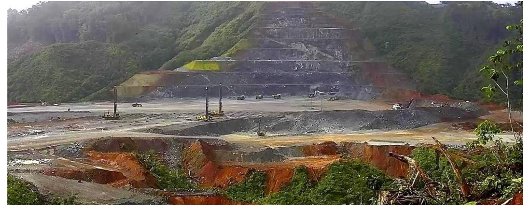
Colina Crusher Box Cut Area
